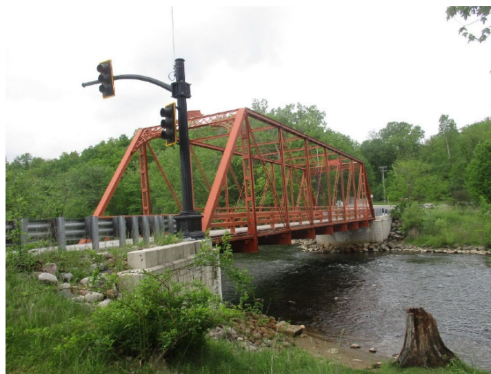
Figure 15: An example of a truss bridge (E. Delhi Road Bridge, over the Huron River (STR 11029), Scio Township)
