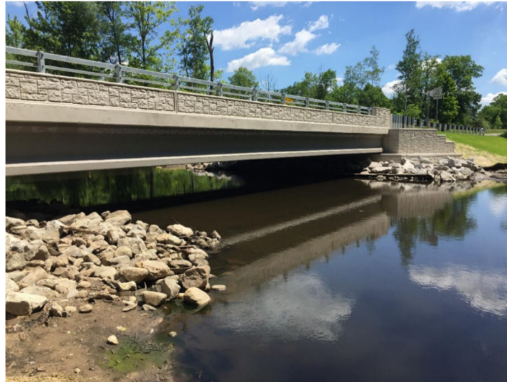
Figure 14: An example of a bridge with concrete beams (Sharon Valley Road Bridge, over River Raisin (STR 10969), Sharon Township)
