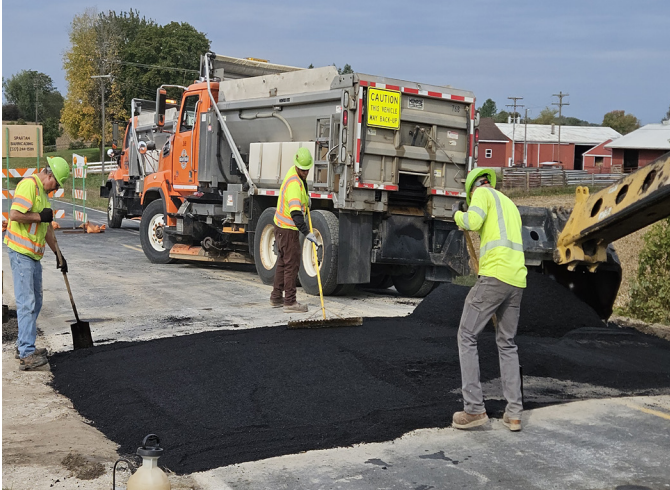
Austin Rd Culvert Replacement (Bridgewater Township)
