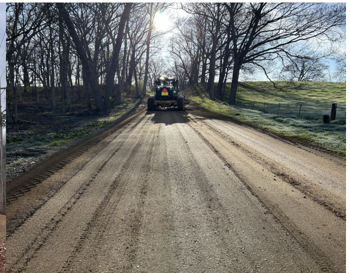
Grading unpaved road
