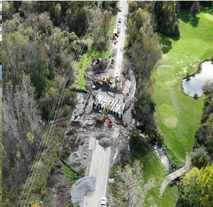
Stony Creek Rd Bridge Replacement (Ypsilanti Township)
