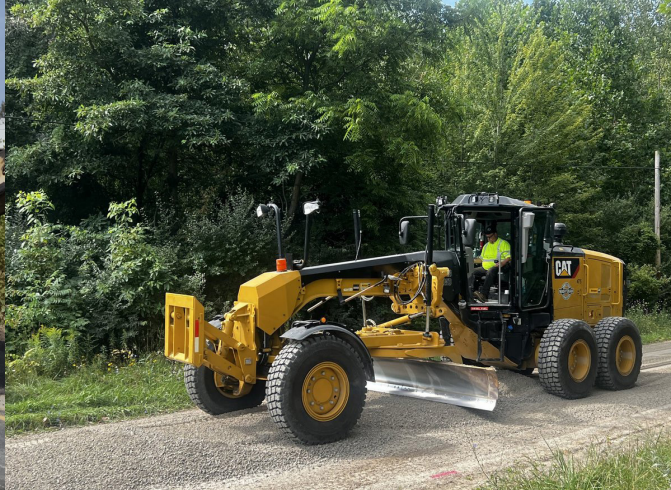
Macy Rd Limestone Resurfacing (Augusta Township)
