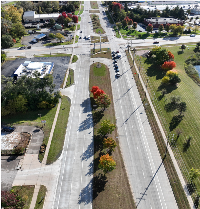
Jackson Rd Concrete Rehabilitation (Scio Township)
