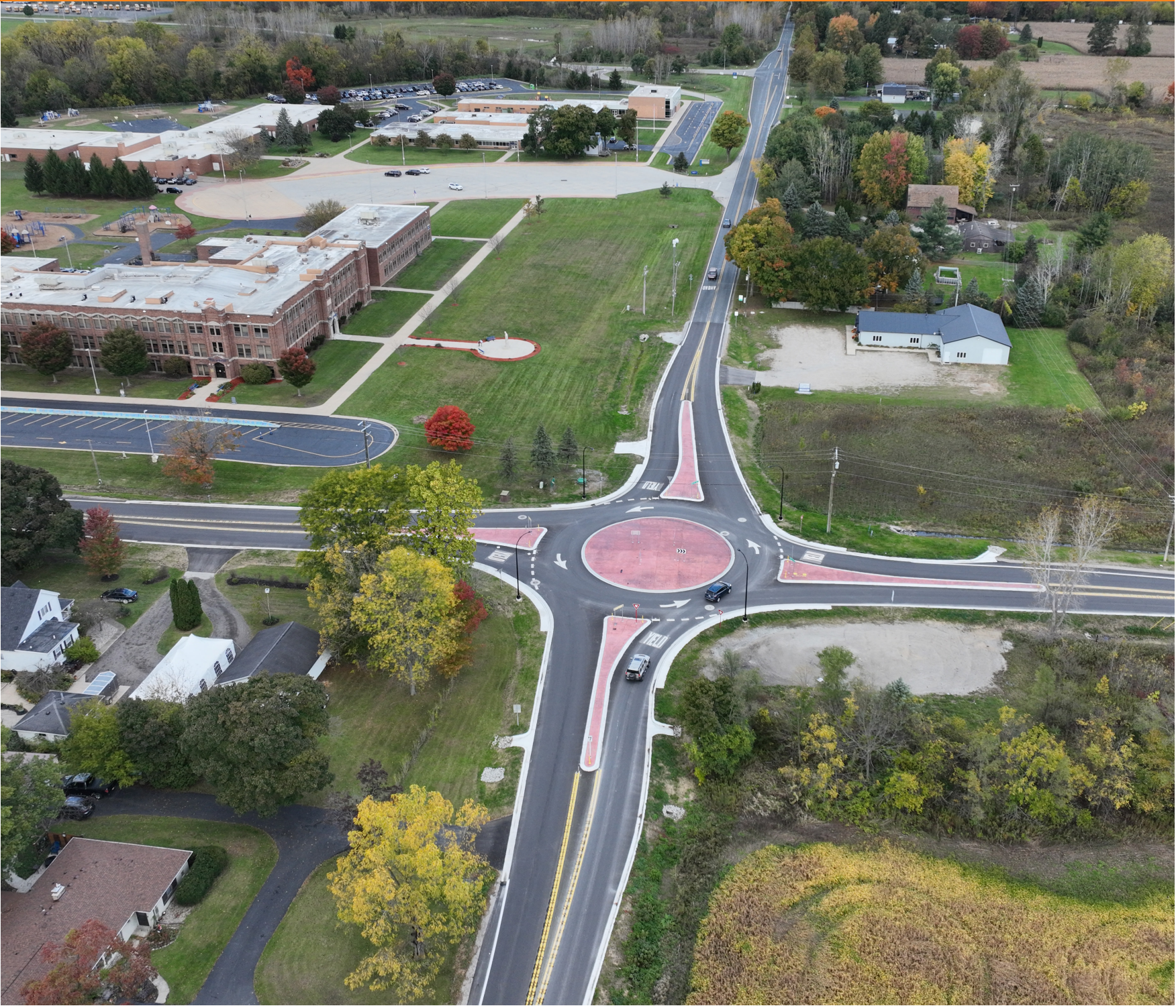
Pictured right is the new Whittaker Rd and Willis Rd Roundabout constructed in Augusta Township.
